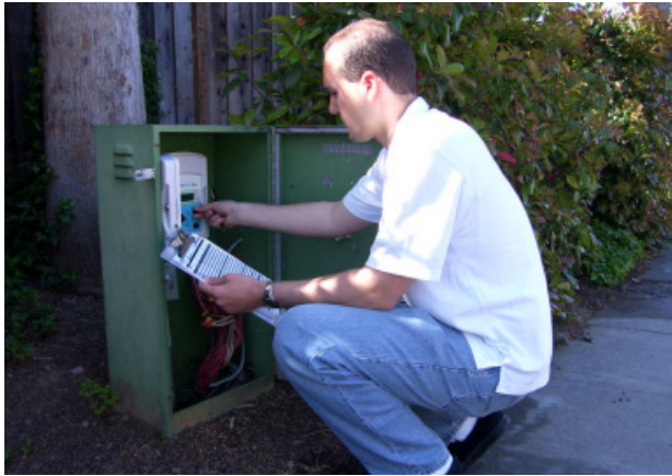
Staff programming an irrigation controller
