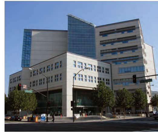
The new Martin Luther King Jr. Library in San Jose is dual-plumbed to use recycled water for all toilet flushing.
