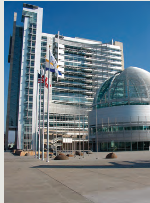
New San Jose City Hall with dual plumbing and ornamental fountain designed to utilize recycled water, starting in early 2006.
