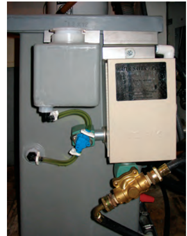
Example of a water conservation device designed to be used with medical x-ray film processors.
