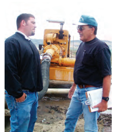
Contractor and District staff discuss booster pump (in background).
