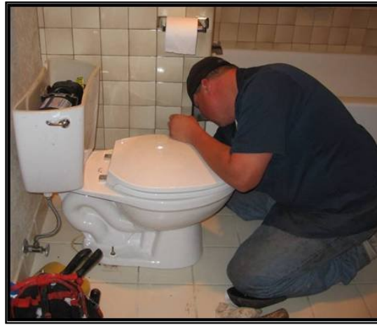
Fixture Replacement Program
