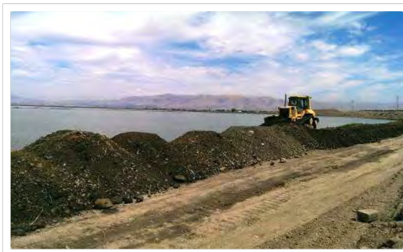
District crews placing sediment at Pond A8
