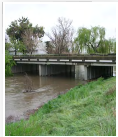
Existing Charcot Road Bridge over Coyote Creek
