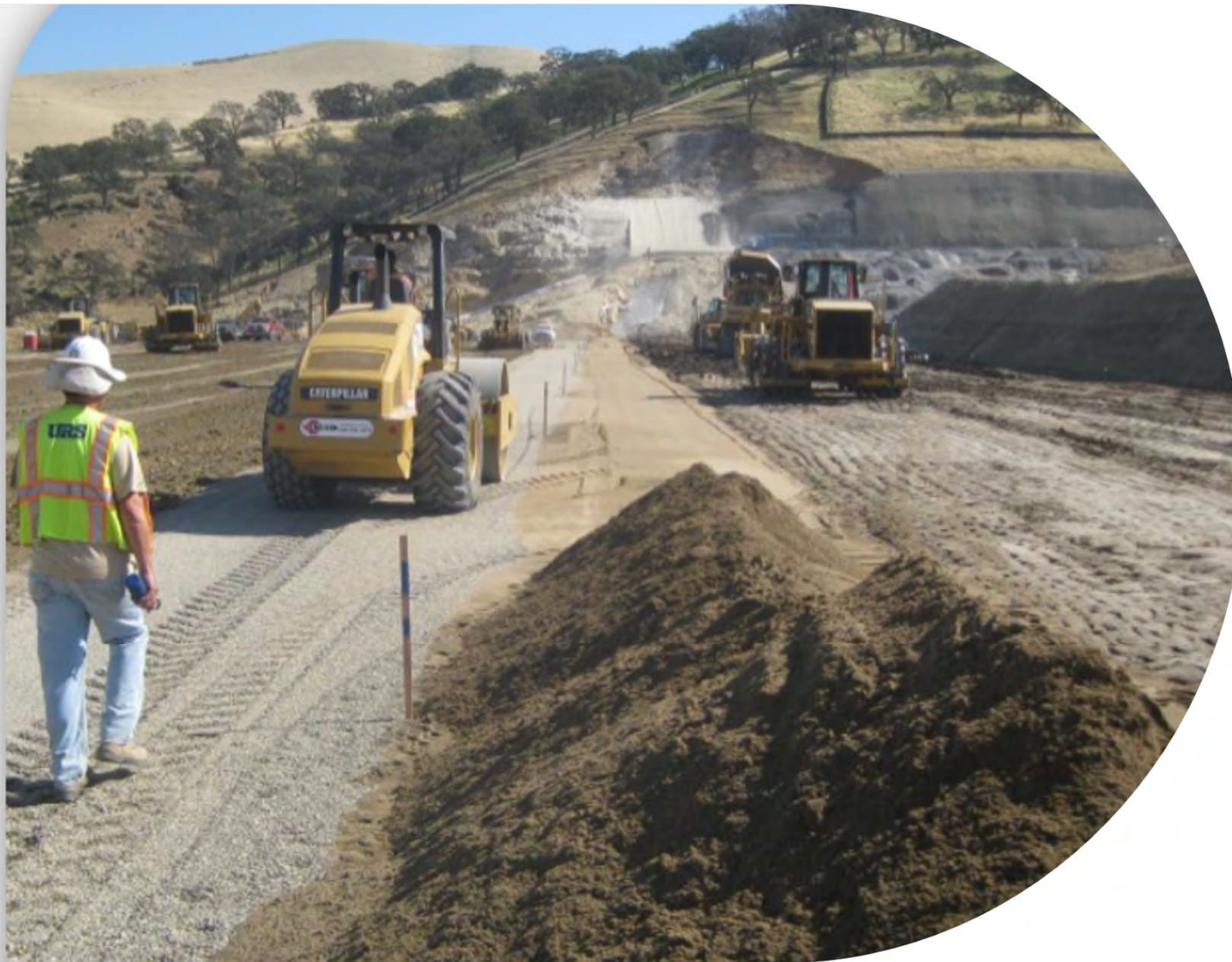
Pictured above: Earthfill Dam Construction in Bay Area
