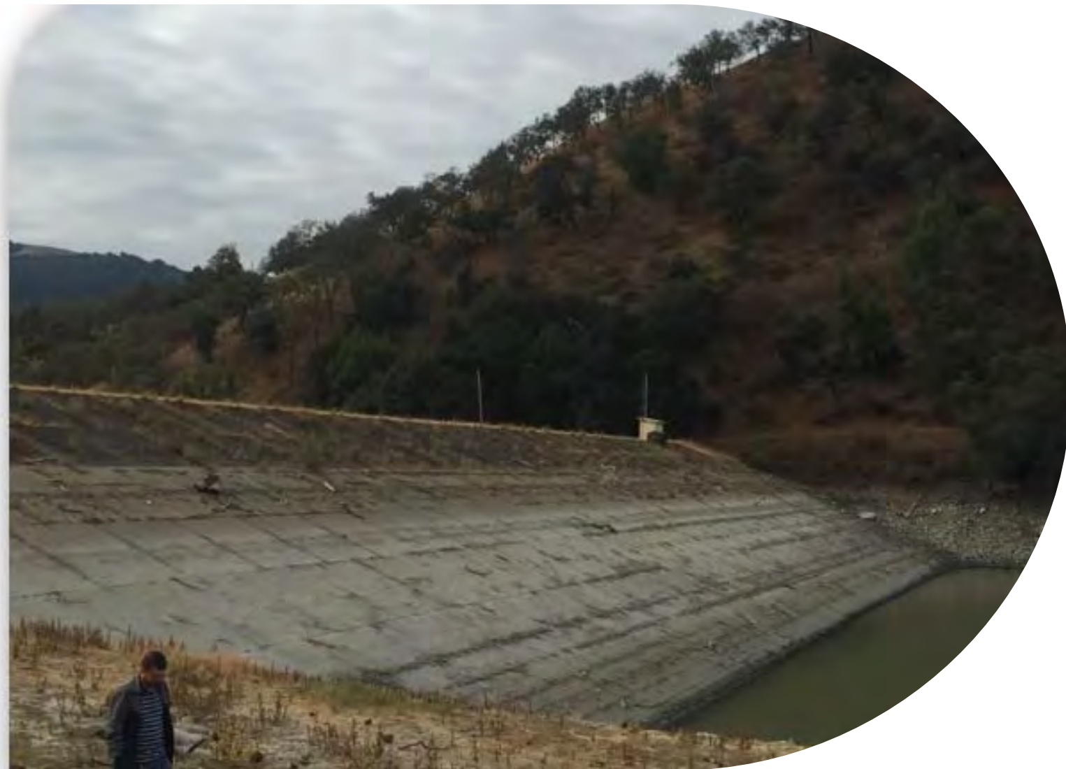
Pictured above: Existing North Fork Dam constructed in 1939
