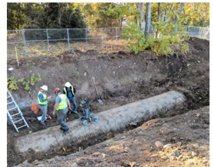
Inspection of Cross Valley and Calero Pipeline.
