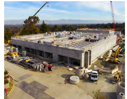
RWTP Reliability Improvement.
