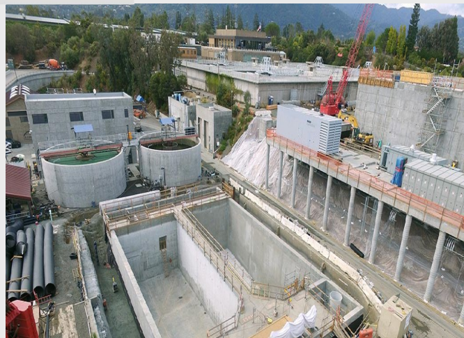
RWTP Reliability Improvements $98 Million ($295 Million Total Cost)
