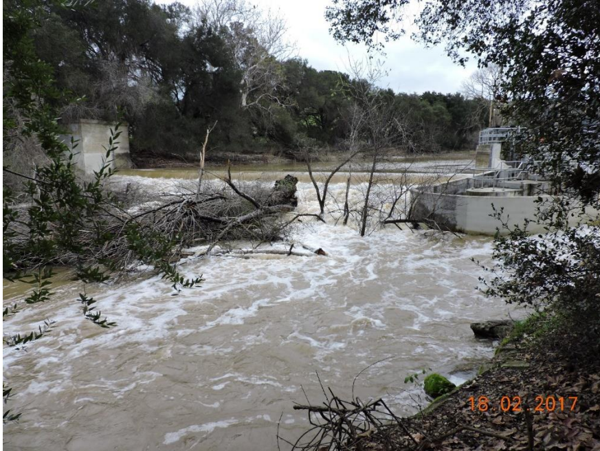
Photo 1. Metcalf Pond dam on 18 February 2017 at 1300 cfs. Radial gates were open and the fish ladder was not passable.
