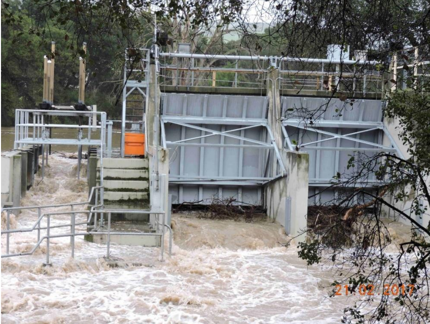
Photo 3. Metcalf Pond ladder and radial gates on 21 February 2017 at 6500+ cfs. The pond water level was high enough that even with the dam panels down there was potential passage in the fish ladder.
