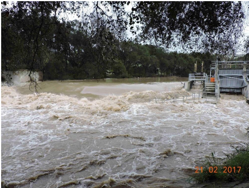
Photo 2. Metcalf Pond dam on 21 February 2017 at 6500+ cfs. Very turbid water from storm flows that filled and spilled from Anderson Reservoir.
