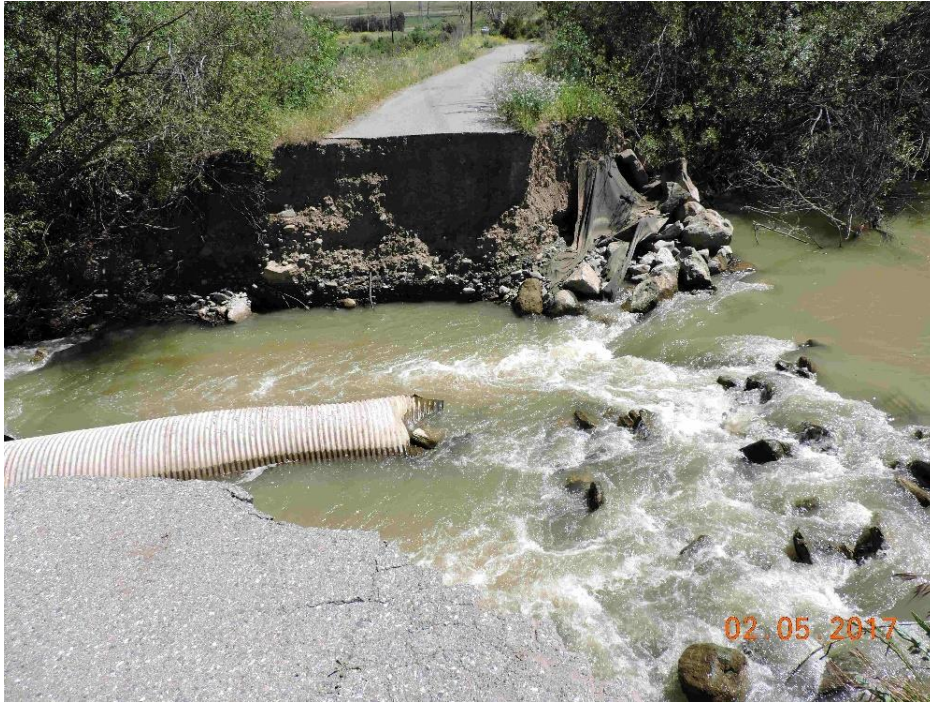
Photo 16. Washed out road and culvert immediately downstream of Ogier Pond #1 on 2 May 2017 at approximately 150 cfs. Stream flow was still turbid (16 cm visibility) from storm water stored in Anderson Reservoir. Visibility had cleared to 75 cm by 26 October 2017.
