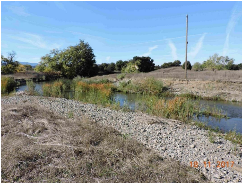
Photo 17. Outlet to Ogier Pond #4 on 18 November 2017 at approximately 70 cfs. The narrow outlet was widened from about 25 feet to 85 feet (including 45 feet above the present water surface).
