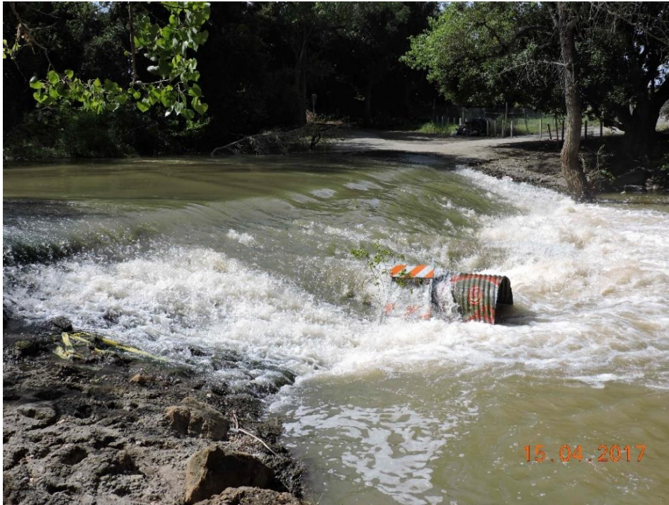
Photo 11. Singleton Road at approximately 450 cfs on 15 April 2017, impassable due to high velocity in the culverts and on the inclined apron.
