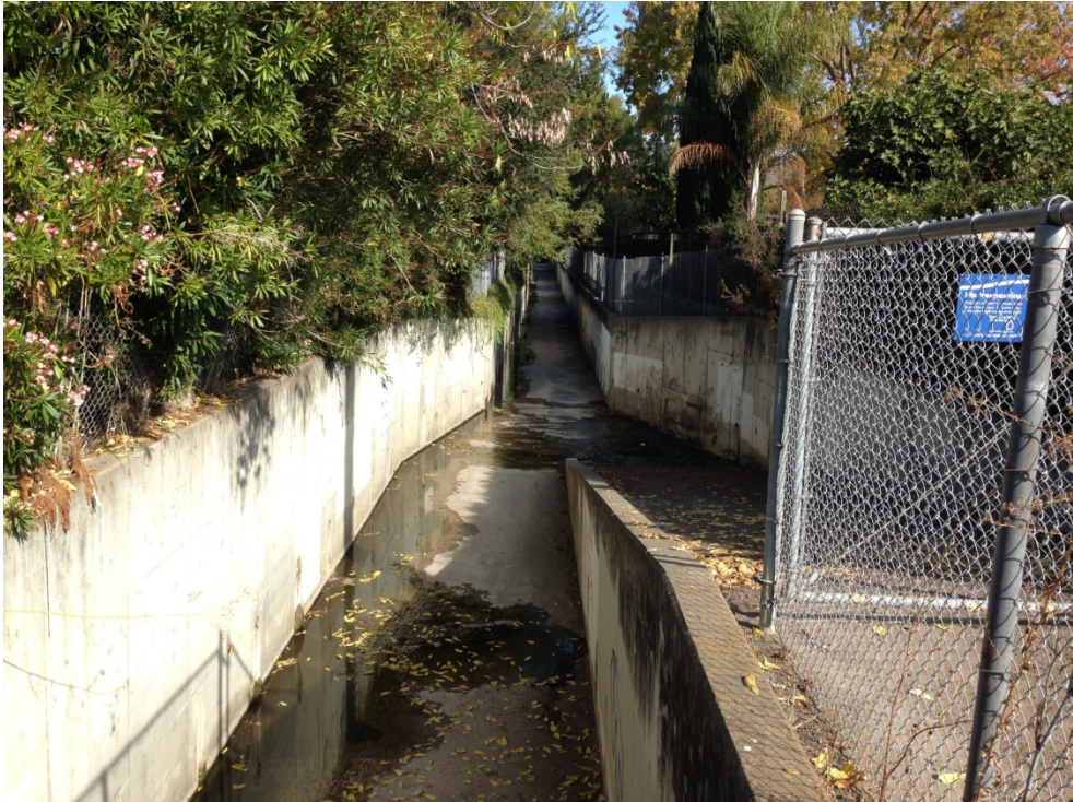
Figure 59. Permanente Creek, Downstream of San Louis Ave
