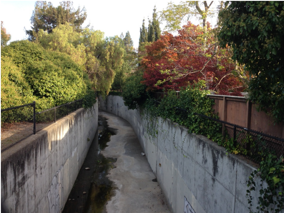
Figure 54. Adobe Creek, Downstream of Alma St
