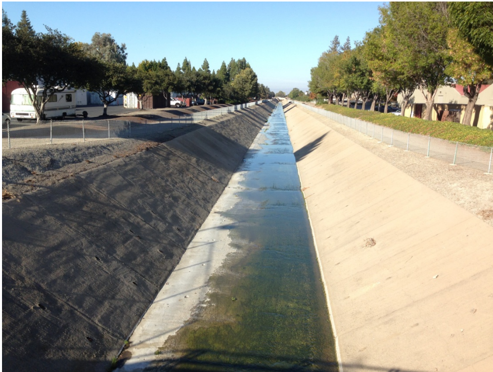
Figure 69. Calabazas Creek, Downstream of E Arques Ave
