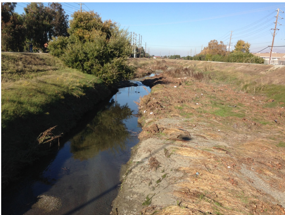
Figure 72. San Tomas Aquino Creek, Downstream of Agnew Rd
