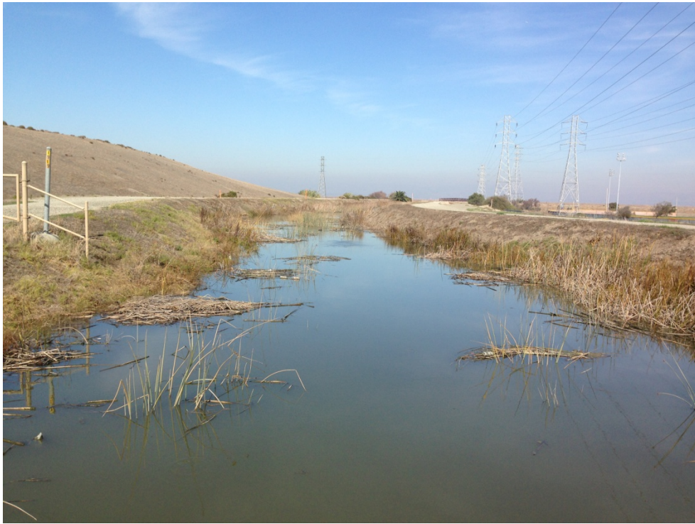
Figure 65. Sunnyvale West Channel, Downstream of W Caribbean Dr
