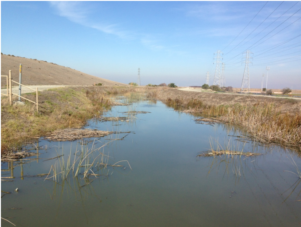
Figure 67. Sunnyvale East Channel, Downstream of E Caribbean Dr
