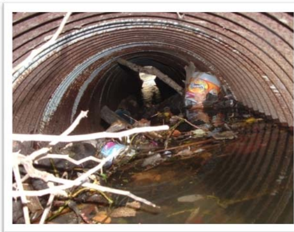
Photographs C-F. C) Side view of Singleton Road culverts, D) Top view of Singleton Road culverts, E) Debris blockage located in left culvert (looking downstream) F) Singleton Road during a high flow event, February 2003.
