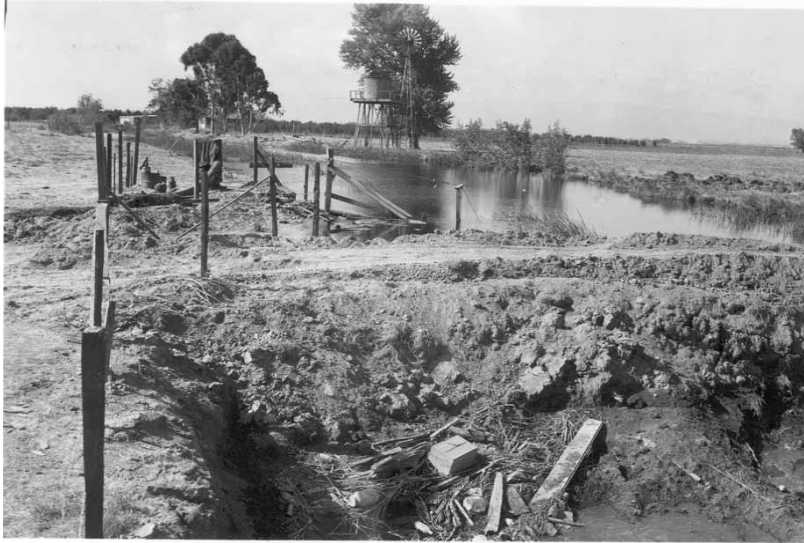
Figure 2. Photograph from May 18, 1932 depicting the original Standish Dam which was constructed as an earthen, wood barrier to prevent salt water intrusion to crops. (SCVWD, 2003).
