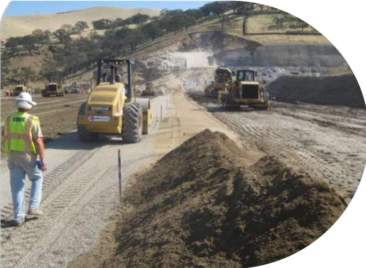
Pictured above: Earthfill Dam Construction in Bay Area
