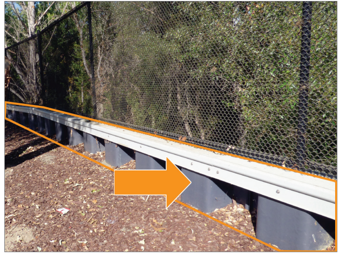
Rocksprings Temporary Floodwall
