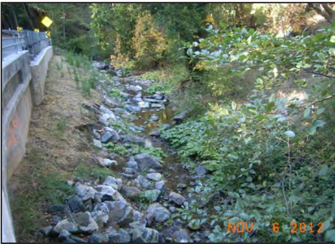
Photo 3. Stevens Creek at Station 931+46.
