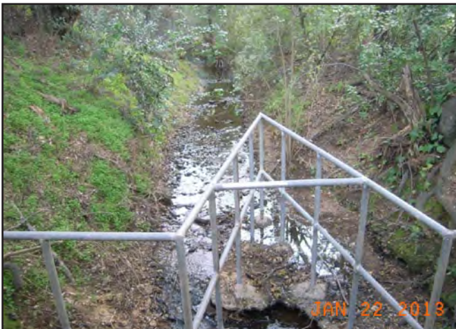
Photo 5. Smith Creek at Station 71+25.
