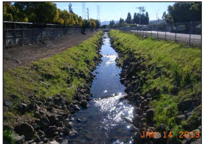
Photo 6. Sunnyvale East Channel at Station 156+28.
