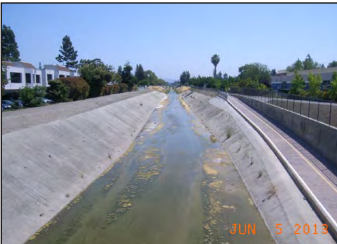
Photo 5. San Tomas Creek at Station 174+17.
