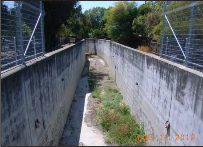
Photo 1. Adobe Creek at Station 219+16.
