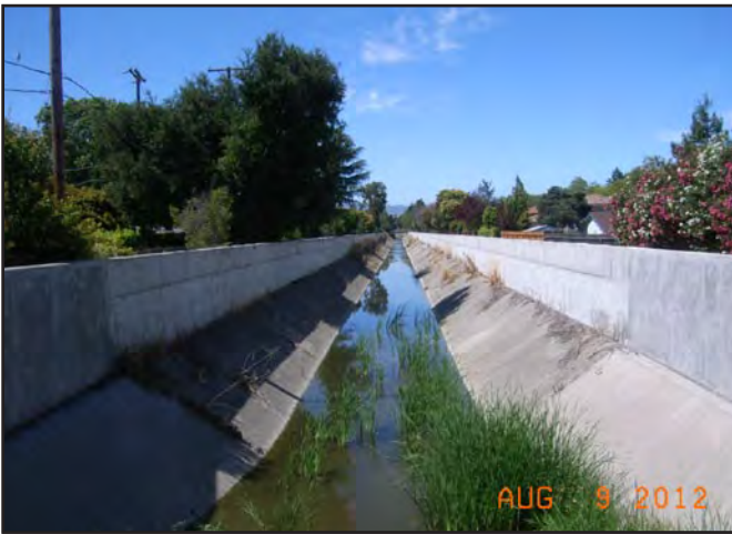
Photo 3. Matadero Creek at Station 121+08.
