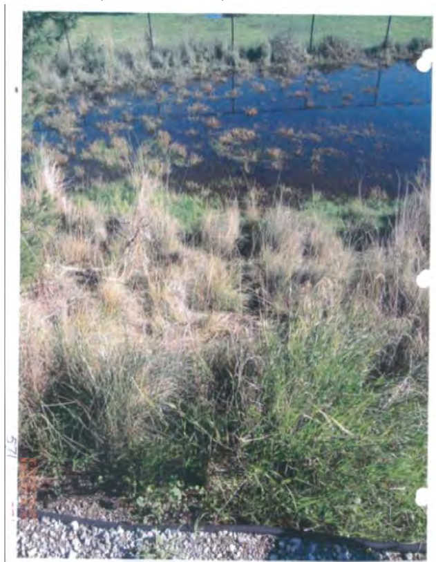
Standing Water (SCVWD 571) – 12/27/2012
