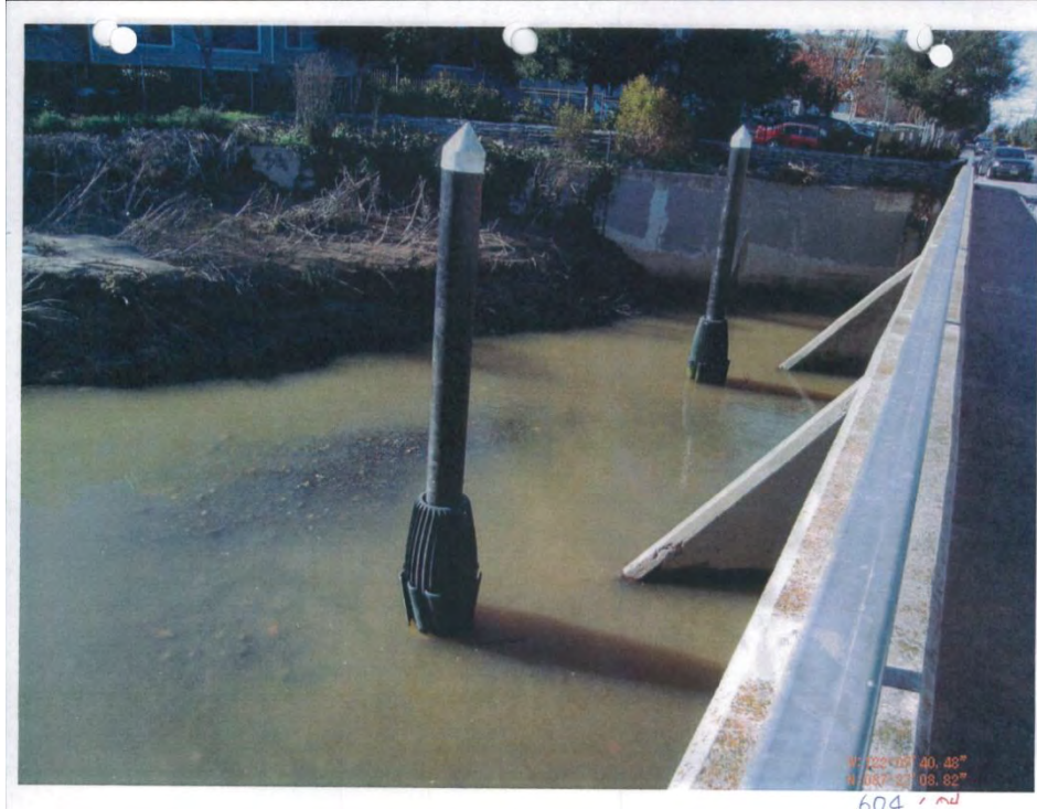
Bridge Shark (SCVWD 604) – 12/31/2012
