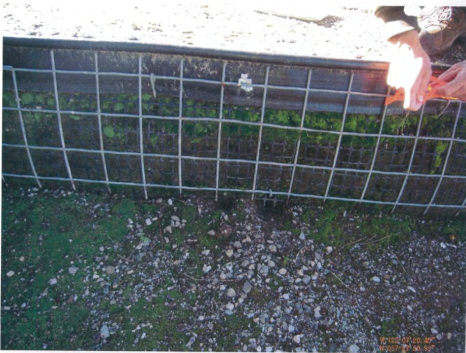
Hole with seepage at lift (SCVWD 573) – 12/27/2012
