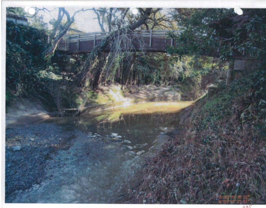
Pedestrian bridge (SCVWD 635) – 12/31/2012
