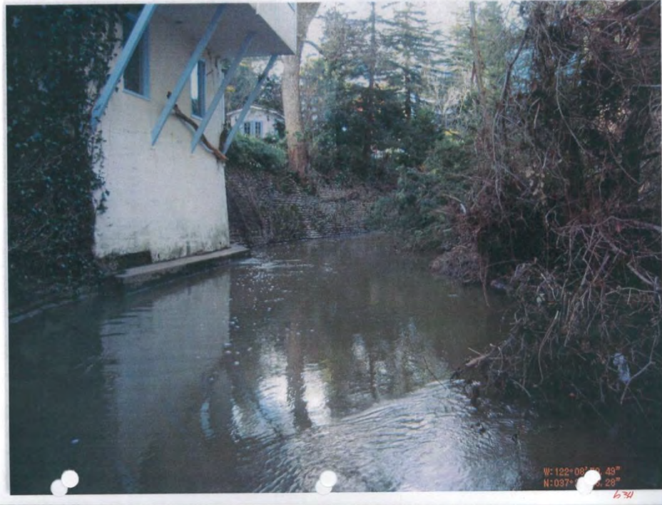
Cantilever house on Lincoln Avenue (SCVWD 634) – 12/31/2012
