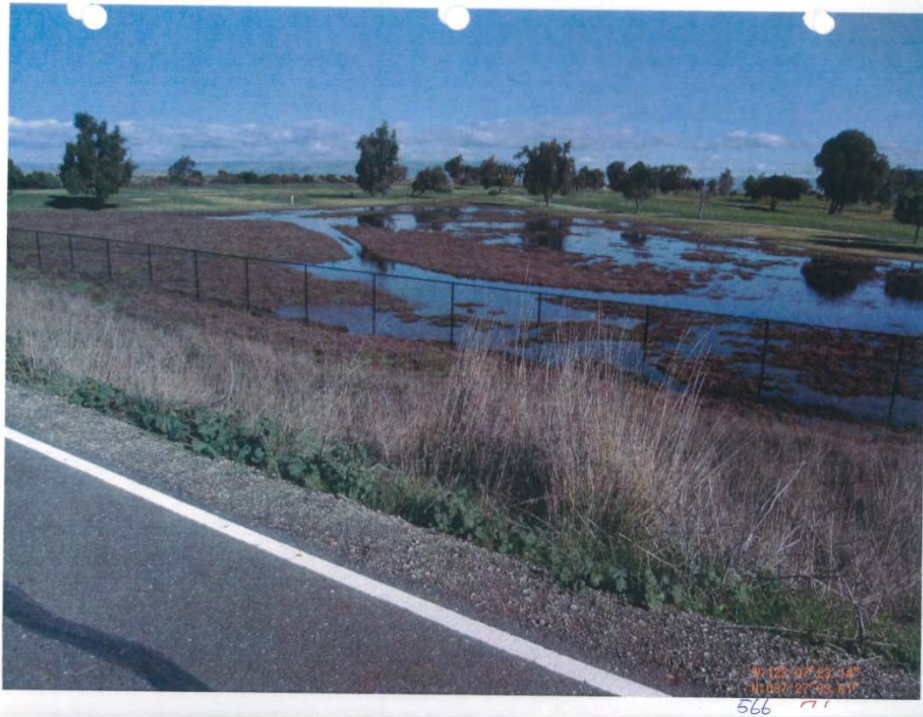
Standing water (SCVWD 566) – 12/27/2012
