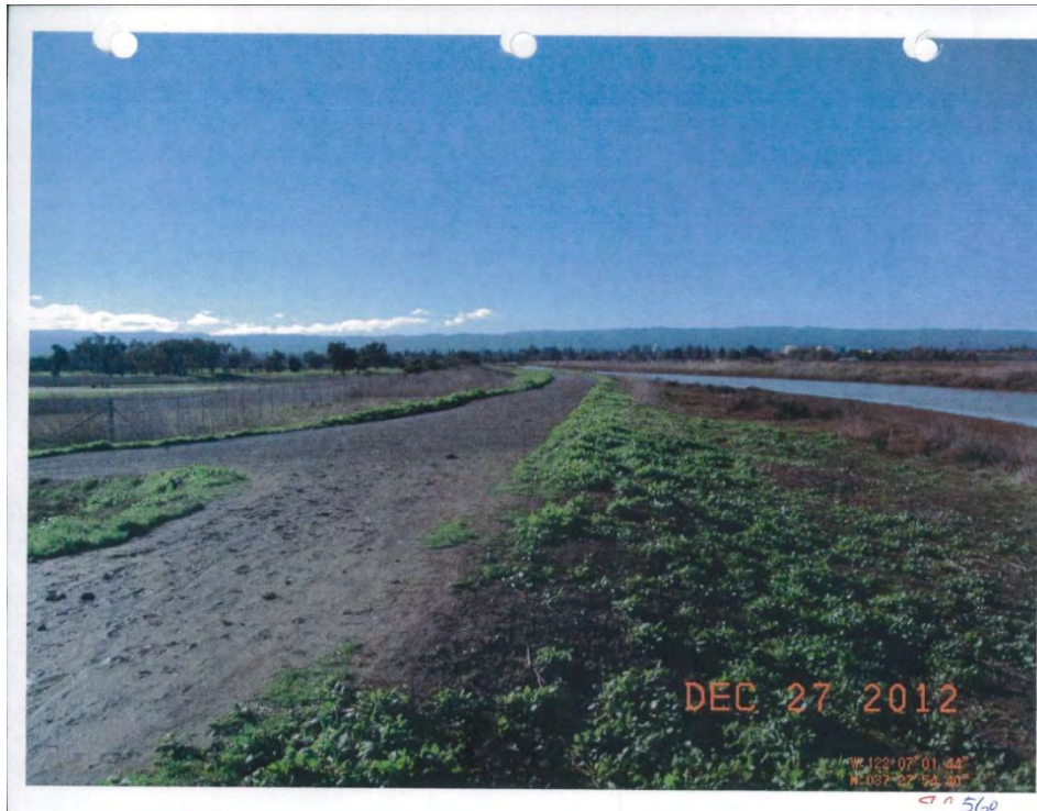
Typical levee (SCVWD 560) - 12/27/2012
