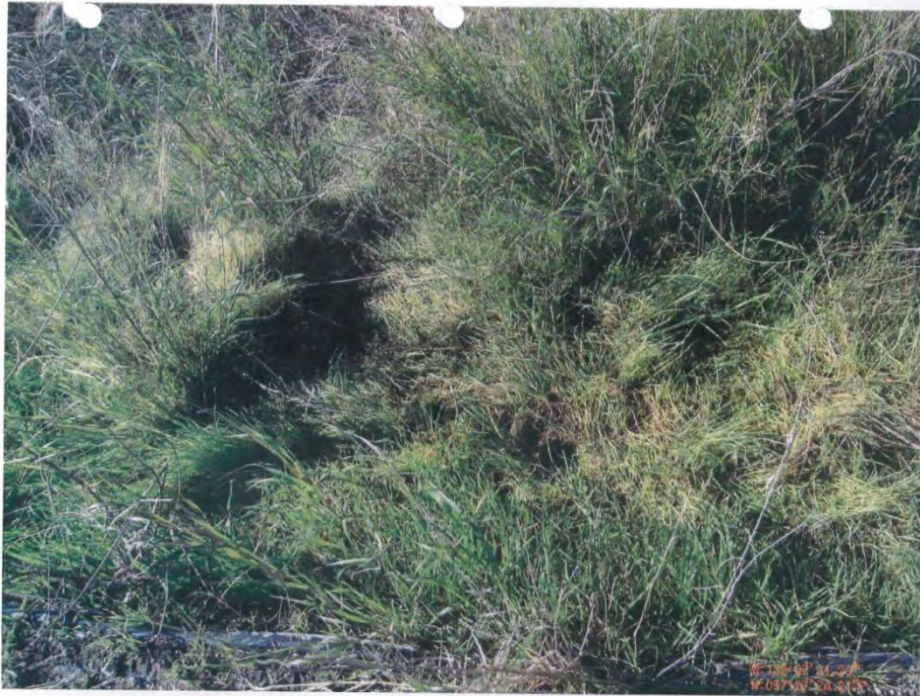
Hole with seepage at lift (SCVWD 572) – 12/27/2012
