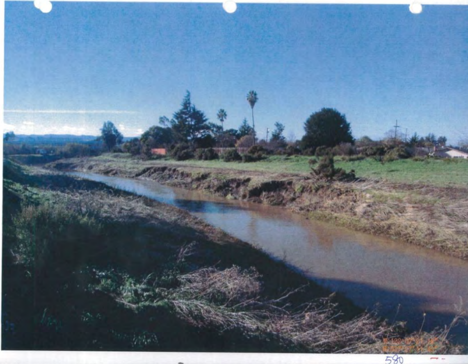
New sloughing on opposite bank (SCVWD 580) – 12/27/2012
