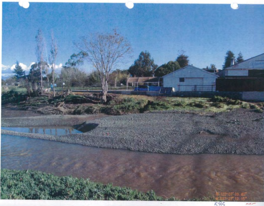
Sediment buildup downstream of Bayshore Road (SCVWD 585) – 12/27/2012
