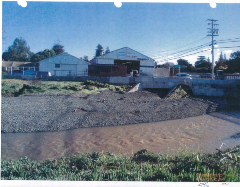
Sediment buildup downstream of Bayshore Road (SCVWD 586) – 12/27/2012
