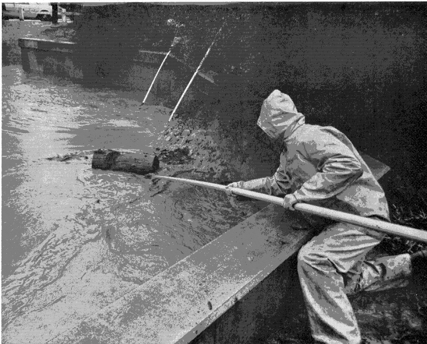
Surcharged culvert on San Francisquito Creek at Chaucer Street.
