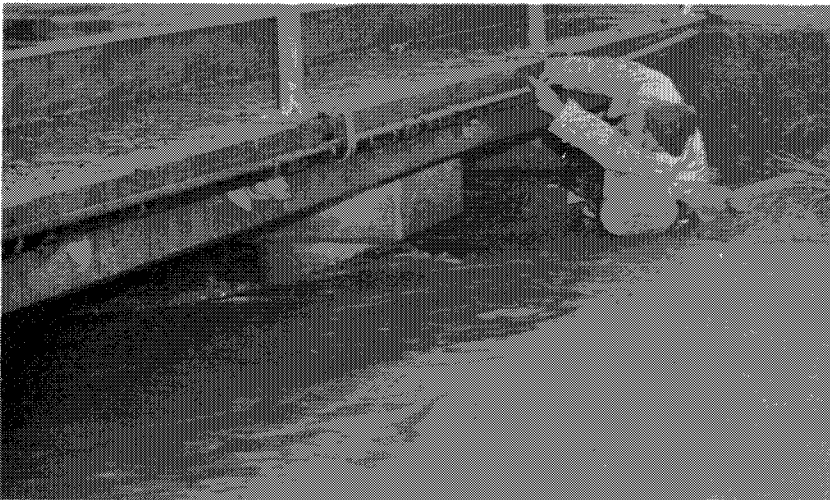
Miller Slough bridge at Church Street in City of Gilroy.
